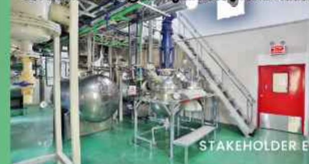
Our manufacturing facility in Hosur, Tamil Nadu
